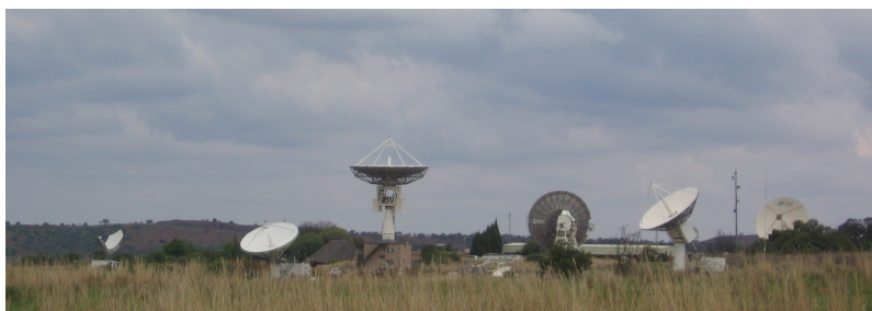
Слика6.4: The CSIR Satellite Applications Center at Hartbeeshoek near Johannesburg. Special antennae track satellites as they pass overhead and download images using radio waves.
