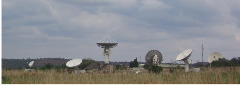
Abb. 6.4: The CSIR Satellite Applications Center at Hartebeeshoek near Johannesburg. Special antennae track satellites as they pass overhead and download images using radio waves.
