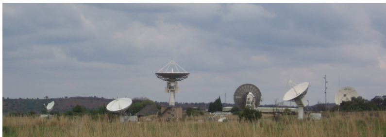
图 6.4: The CSIR Satellite Applications Center at Hartebeeshoek near Johannesburg. Special antennae track satellites as they pass overhead and download images using radio waves.
