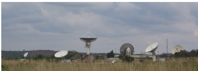
Fig. 6.4: The CSIR Satellite Applications Center at Hartebeeshoek near Johannesburg. Special antennae track satellites as they pass overhead and download images using radio waves.
